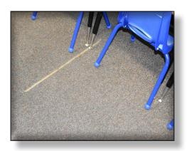
■ Since the carpeting is most likely asbestoscontaining in the three lower-level rooms, environmental testing and potential issues should be factored into the project budget. >
