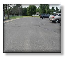
■ The District should reseal the parking lot and repaint the lines to prolong its useful life. Resealing the main lot may be an option to prolong life. The District should also repaint the curbs where the paint has worn off over the past year.
