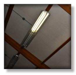
■ Multiple fixtures were broken or missing lights during the walkthrough. The district should replace these fixtures and lights first. ▶
