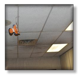
The district should replace the broken tiles as needed and further investigate the root cause of stained ceiling tiles throughout the facility.
