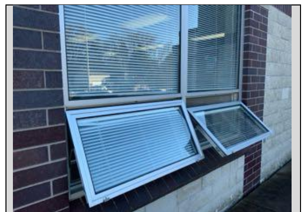
Operable aluminum windows with integral blinds.
