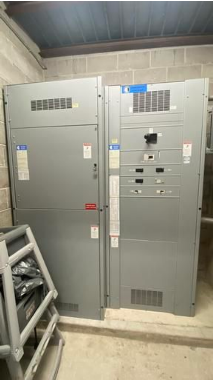
IMG_6810 Added as Reference Taken on Feb 16, 2026, 2:42 PM CST Added on Feb 16, 2026, 2:53 PM CST Added by Daniel Sieben
