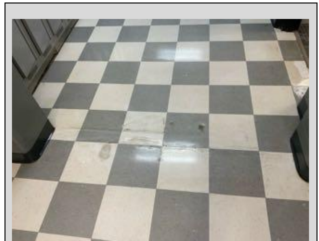
VCT cracking
