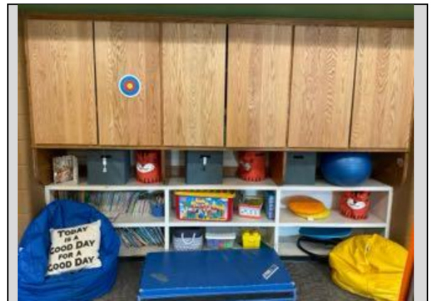
Wood casework with new doors – no handles.
