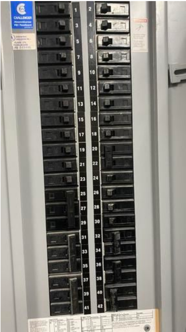
IMG_6820 Added as Reference Taken on Feb 16, 2026, 2:57 PM CST Added on Feb 16, 2026, 2:58 PM CST Added by Daniel Sieben
