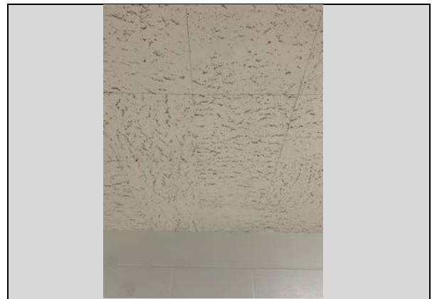
Concealed spline ceiling tiles.
