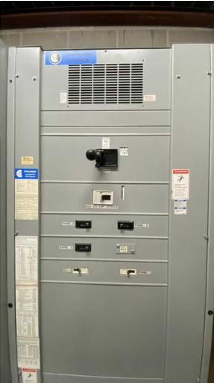
IMG_6811 Added as Reference Taken on Feb 16, 2026, 2:42 PM CST Added on Feb 16, 2026, 2:53 PM CST Added by Daniel Sieben
