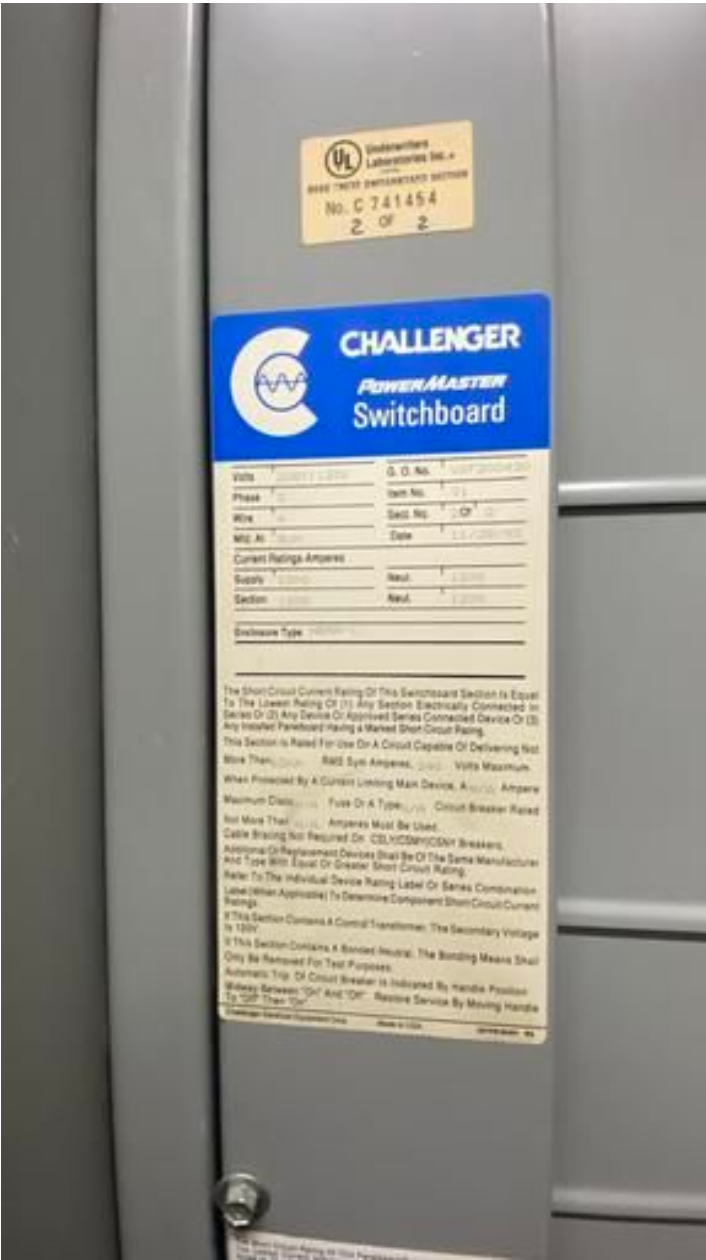
IMG_6812 Added as Reference Taken on Feb 16, 2026, 2:42 PM CST Added on Feb 16, 2026, 2:53 PM CST Added by Daniel Sieben
